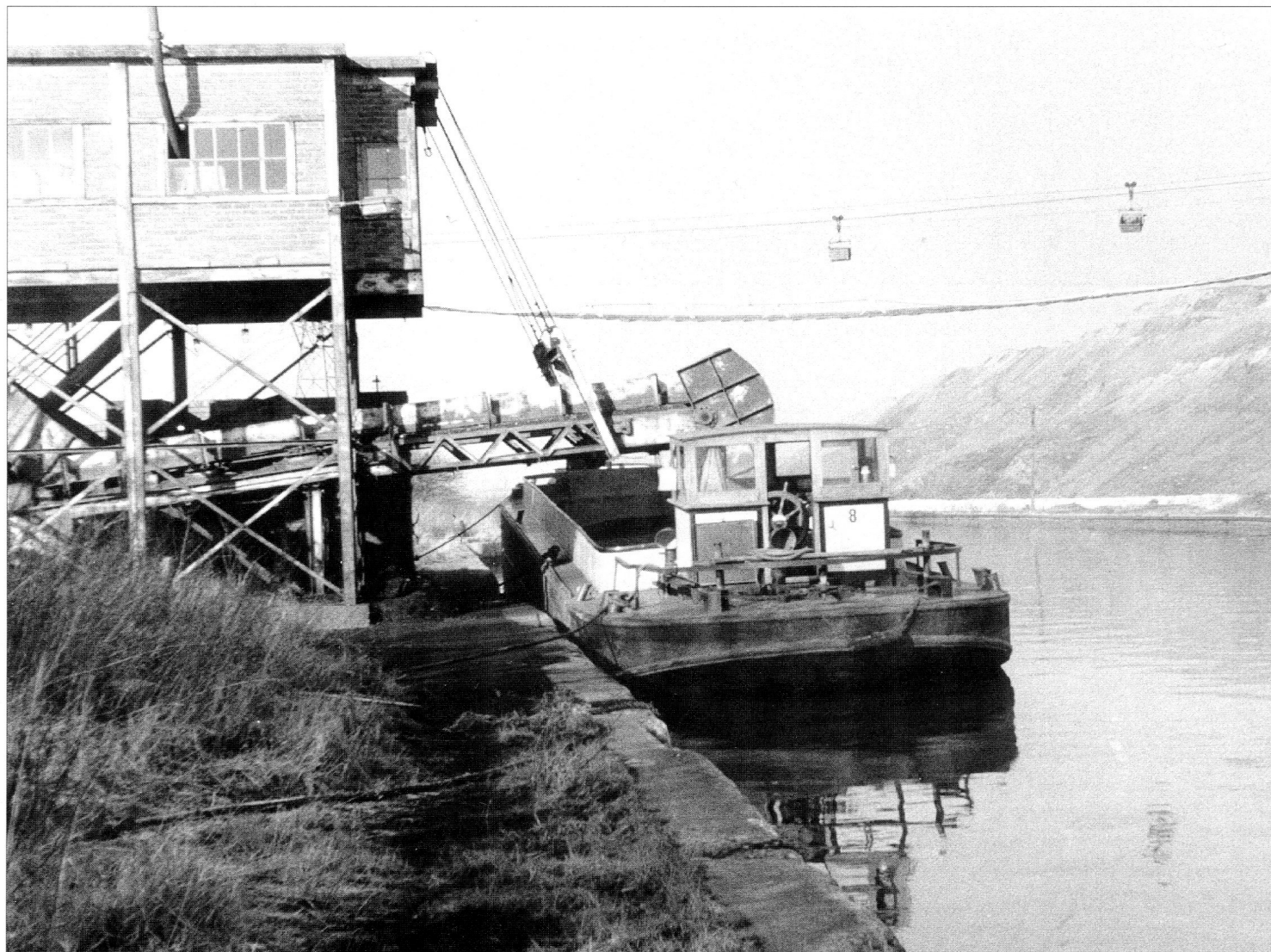
Loading at the canal staith, 6 February 1970. By this time the old method of loading had been superseded by a conveyor belt. In the distance is the aerial ropeway to the tip on the north side of the canal at Swillington Park. Driver Dave Fallowfield considered that the line to the staith was in need of repair but the engineers seemed to turn a deaf ear to his comments. However, on one occasion one of the engineers needed to inspect the staith and he cadged a lift on Dave's engine. Dave made sure that the trip was much faster than usual – the ride was rough enough to frighten the living daylight out of the engineer and the track was attended to very shortly afterwards! PHOTOGRAPH: KEITH TAYLORSON; THE TRANSPORT TREASURY
