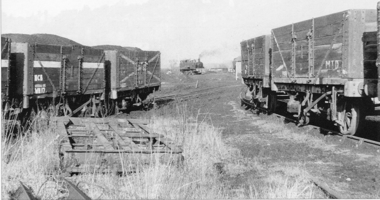
Quiet days at a once busy colliery - this was the herbaceous scene at Water Haigh on 6 February 1970, only a couple of months before it ceased production. PHOTOGRAPH: KEITH TAYLORSON; THE TRANSPORT TREASURY
